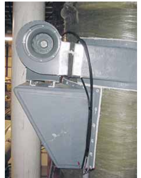
When selecting pumps and blowers, refer to the motor specifications and select those with low dB noise levels. Also, all pumps and blowers should be installed using vibration-isolating motor mounts, and vibration transmission from pumps or regenerative blowers to connecting plumbing may be lessened through the use of expansion couplings.
