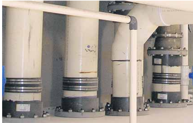
When selecting pumps and blowers, refer to the motor specifications and select those with low dB noise levels. Also, all pumps and blowers should be installed using vibration-isolating motor mounts, and vibration transmission from pumps or regenerative blowers to connecting plumbing may be lessened through the use of expansion couplings.
