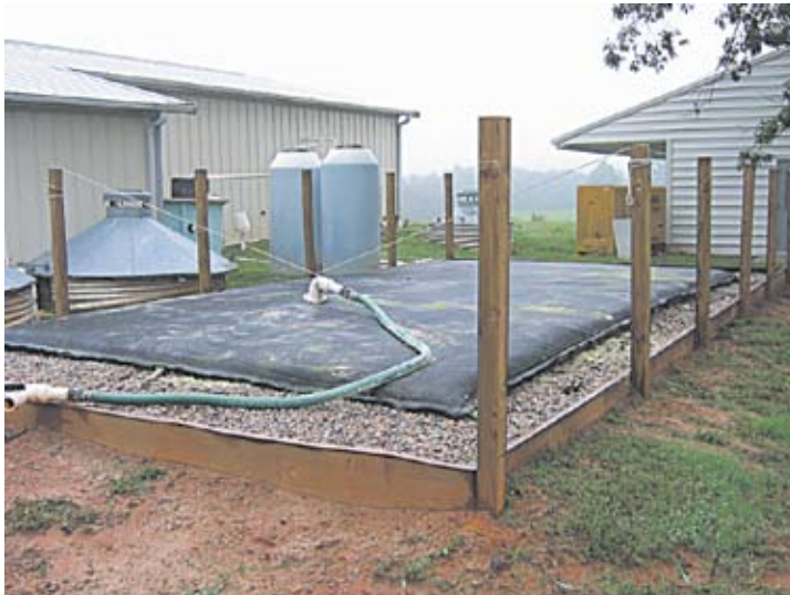
Geotextile bag used for collecting waste solids at North Carolina State University (Photo courtesy James Ebeling)
