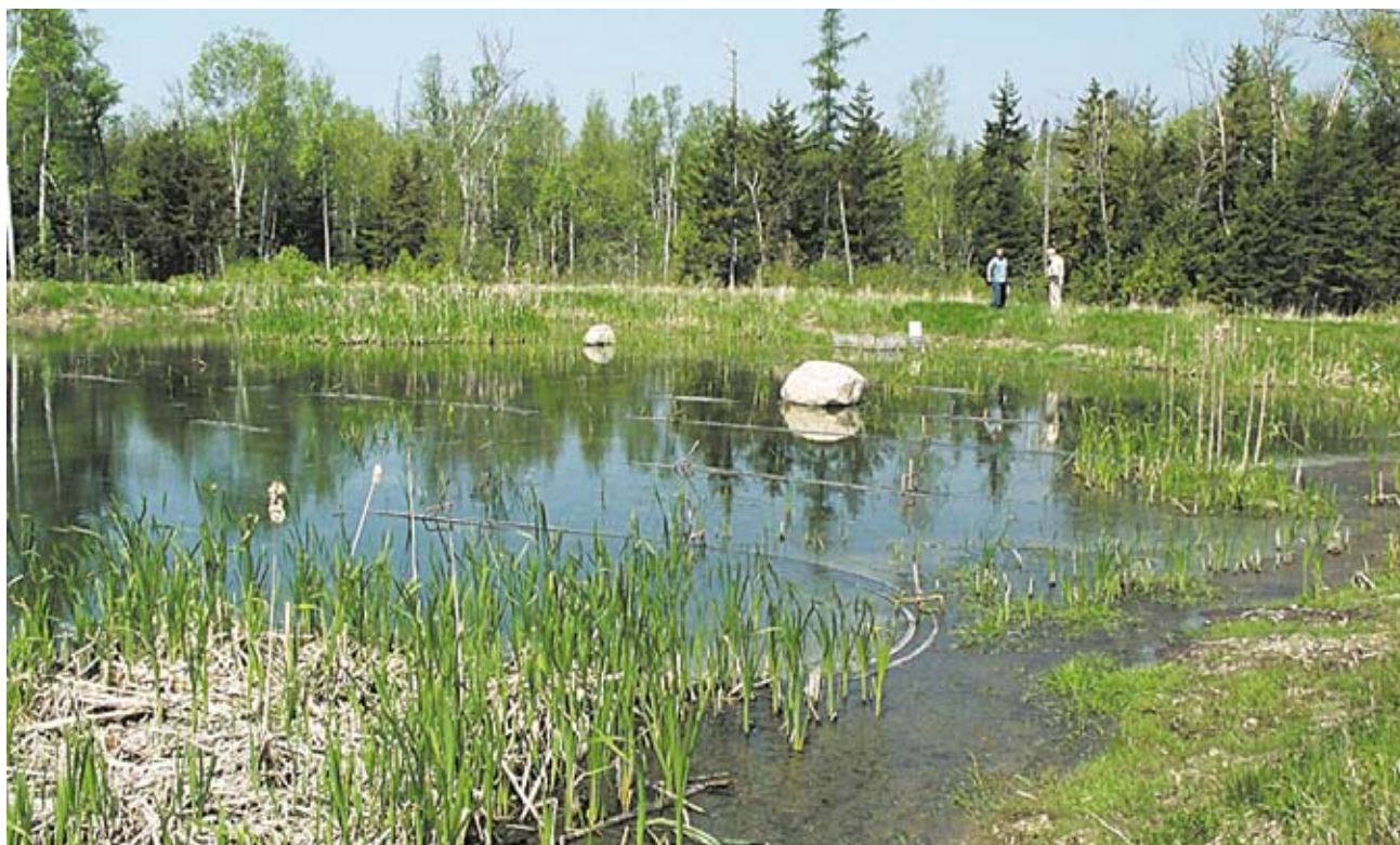
Designed wetland. Wastewater is discharged to a small stream near where the observers are standing (file photo).
