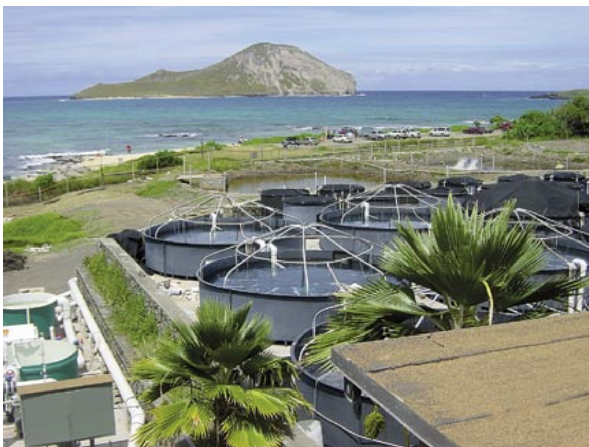
PRAqua-designed Land-based recirculating seawater facility for raising Amberjack at Oceanic Institute. The water treatment system is on the left.
