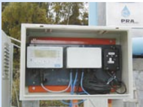
A Point Four PT4 system monitor at a recirculation facility in Chile.
