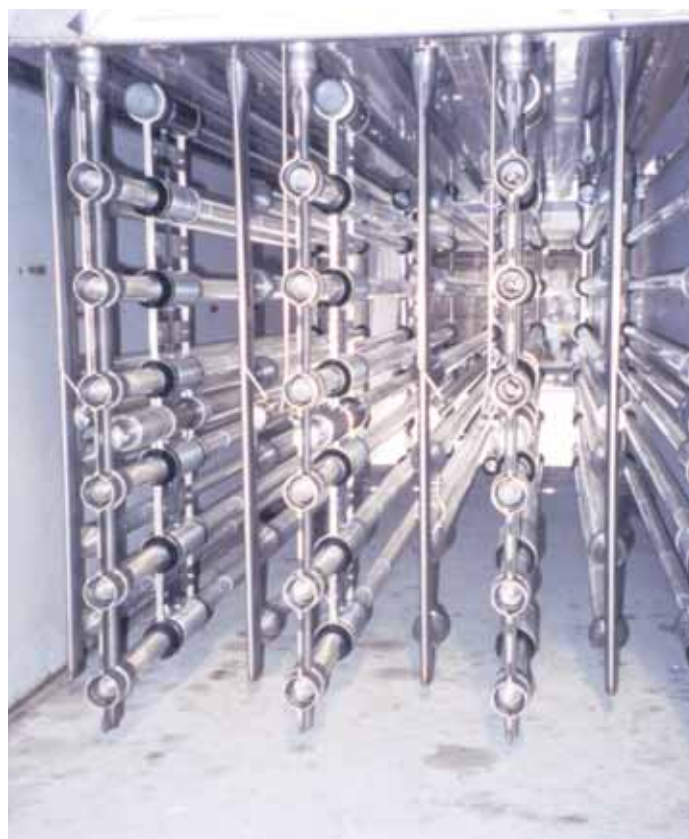
Large, Trojan open channel UV system. Usually used for very large flow systems.
